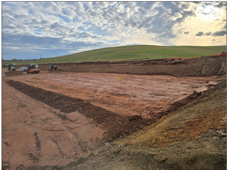
Photo No. 11 Completed clay liner for the test pad.
