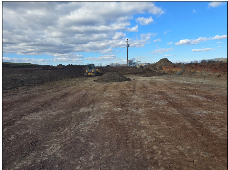
Photo No. 8 Preparing subgrade surface for the construction of the test pad.
