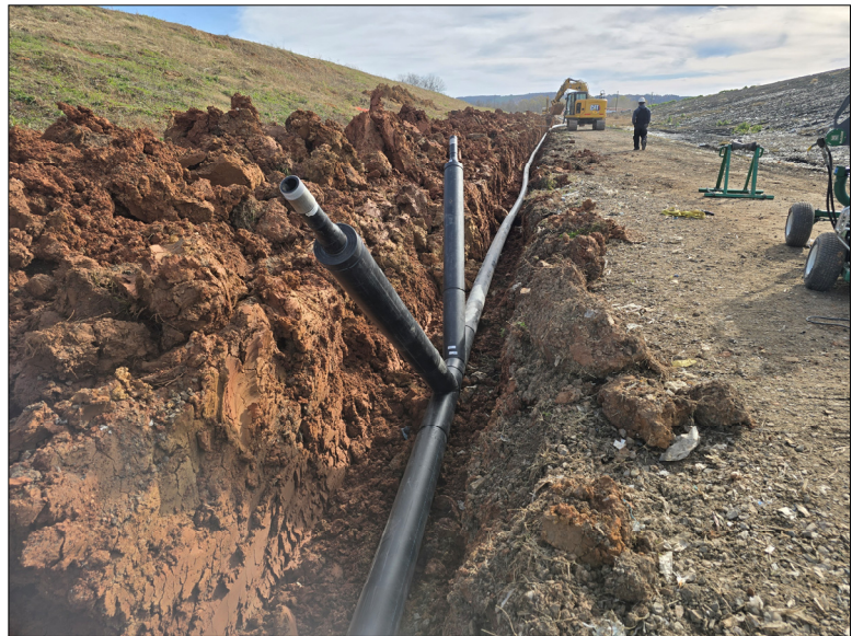
Photo No. 5 Installation of the 8" x 4" HDPE leachate forcemain and the leachate cleanout on the east side of Cell 5.
