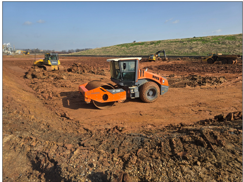
Photo No. 14 Grading and compacting the clay liner.
