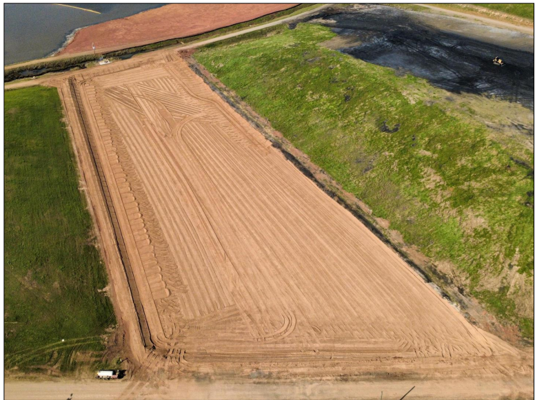
Photo No. 20 Completion of the protective cover.
