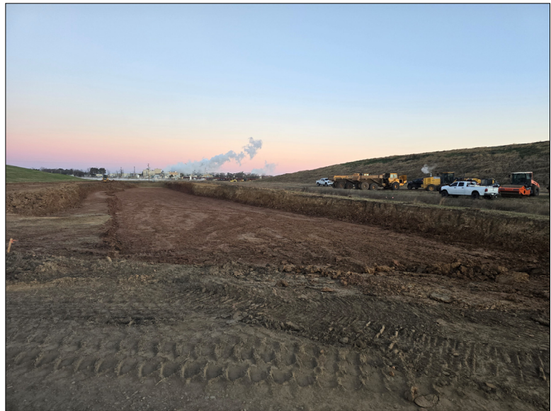
Photo No. 2 Utilizing a dozer, excavator, and haul trucks to excavate cell construction area. Soil was hauled to a stockpile south of the existing closed landfill.
